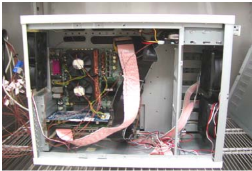
The view of the thermocouples connections.
